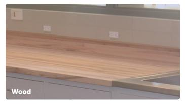
Thickness can be specified based on aesthetic preference or function. Common options range from  $1.25^{\circ} - 2^{\circ}$ . Also, the top finish can vary from a natural surface with an applied oil that can be reapplied as needed, to a factory applied conversion varnish that will give years of life.
